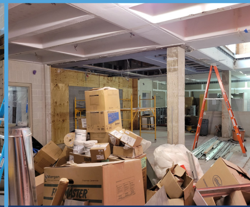
Enclosure complete, starting to install floors, walls and lights – October 2021
