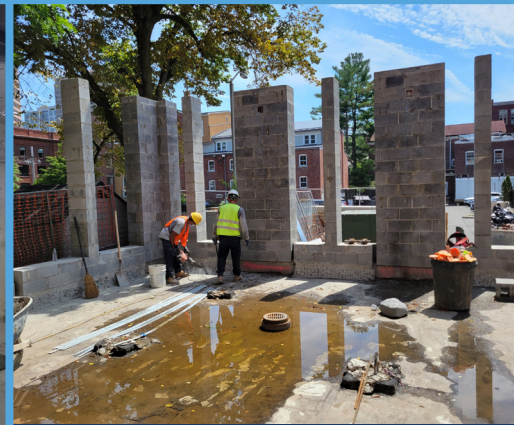
New terrace walls and drains being installed – July 2021
