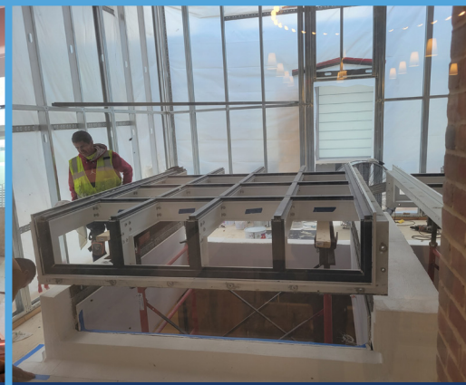
Installing and waterproofing the skylight – April 2022
