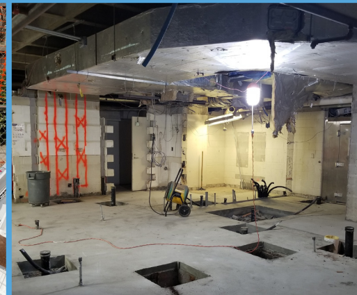
New kitchen concrete slab, with plumbing and electrical runs complete – April 2021
